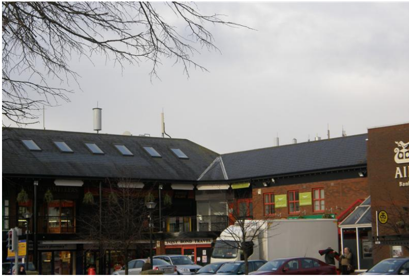
Transmitter Site Photo
